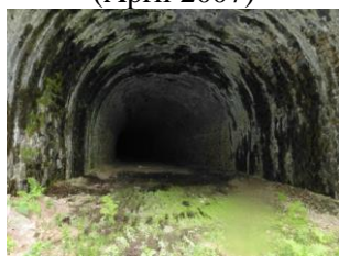
Interior of the Confolent tunnel (May 2015)
