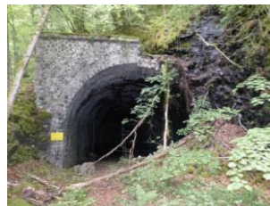
Northern entrance of the Confolent tunnel (May 2015)
