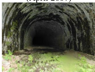
Interior of the Confolent tunnel (May 2015)
