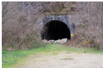
Southern entrance of the Confolent tunnel (April 2007)
